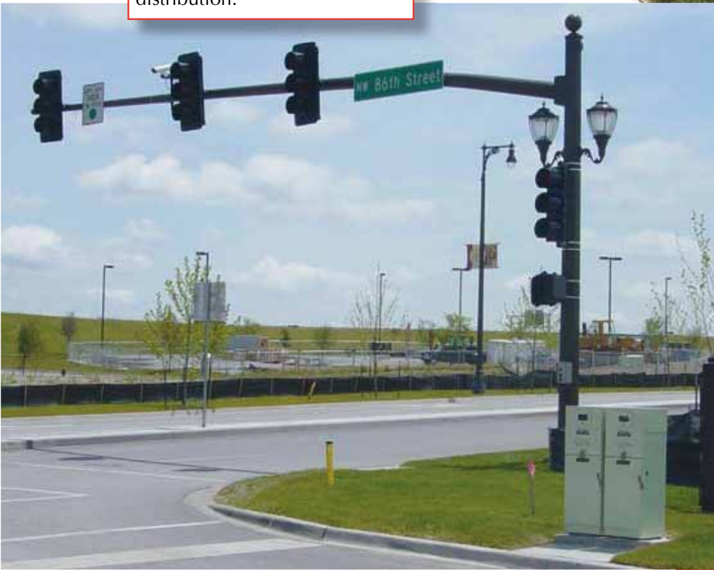
Location: Kansas City, MO Description: Zona Rosa Shopping Center. Multiple pedestal locations throughout shopping area providing street lighting and traffic signal distribution.
