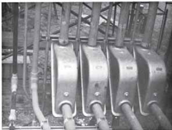
Conduit Systems Installations
