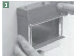
3 Install the second FlameStopper box to opposite side of the wall and tighten all bolts.
