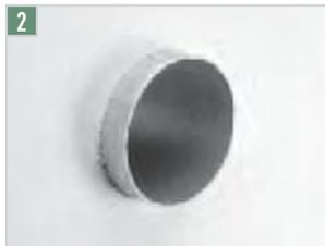
2 Install FlameStopper box to one side of the wall using adhesive strips. Insert the proper length of conduit thru the opening and press in place.
