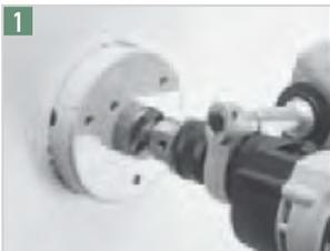
1 Determine the location for the fitting on the wall and cut a hole to fit FlameStopper EMT conduit.
