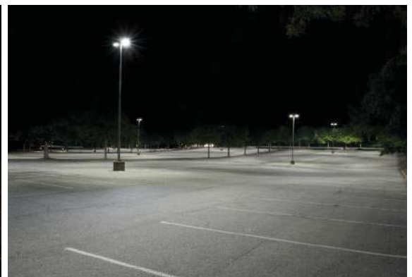
New 210 watt LED, double configuration, mounted at 28 ft.
