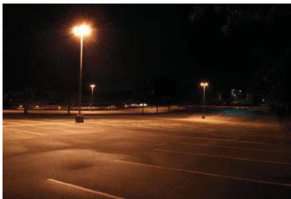
Old 400w HPS units, double configuration, mounted at 28 ft.
