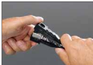
2. Snap Multi-Tap insulators over connectors.
