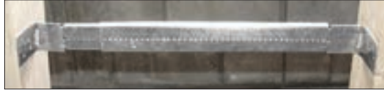
TELESCOPING SCREW GUN BRACKET IN WALL OPENING
