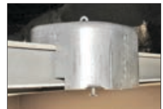
3) Ensure proper fit for ceiling tile.
