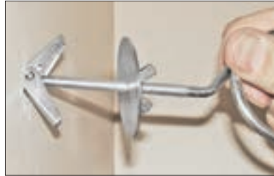
Toggle in...Tighten down
