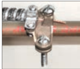
Clamp secures BX/MC in place
