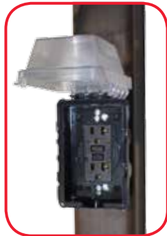
Detail of 120v GFI receptacle with weatherproof cover
