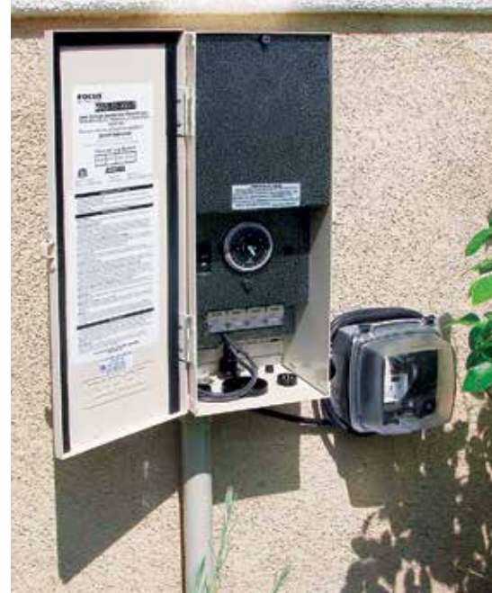
MAS-12-300-T Transformer with Integral Timer Custom Powder Coat Finish
