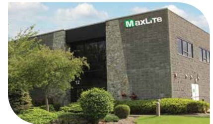
(HQ) West Caldwell, NJ
