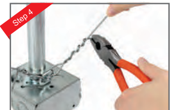
Step 4 Mount seismic wires to surroundings and tie to holes of CLCSL
