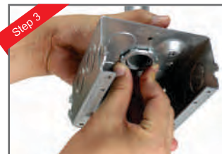
Step 3 Secure conduit to box using locknut
