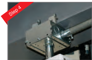
Attach side plate with screws to finish installation
