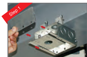
Install EALB with side plate and cover plate removed
