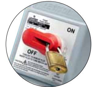
Handle with padlock installed
