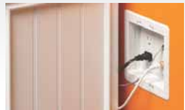
Finished Installed Shot.
