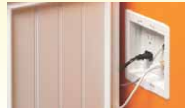
Finished Installed Shot.
