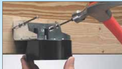
Nails to SINGLE JOIST
