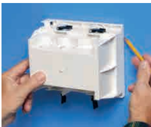
1 Determine box location. Use box (without trim plate) as template for hole.
