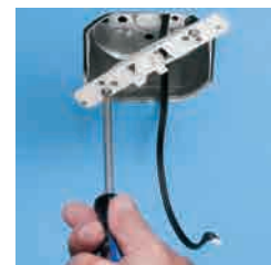
1 Attach SC5 bracket to box.
