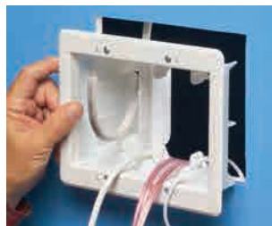
2 Cut drywall. Attach trim plate to box. Install box assembly in opening.
