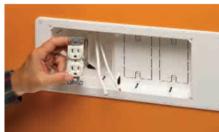
3 Install power and low voltage wiring devices.
