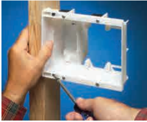
1 Attach box to stud. Note tabs for proper positioning of box for drywall.
