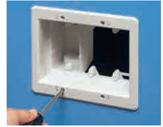
OPTIONAL for new work: Tighten mounting wing screws to pull the box securely against the wallboard and provide added box stability.
