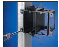
or SCREW onto Metal Stud!
