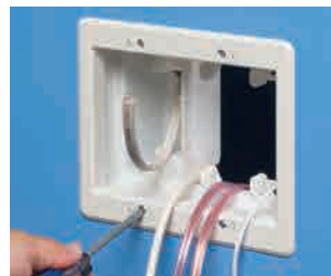
3 Tighten mounting wing screws to pull the box securely against the wallboard.
