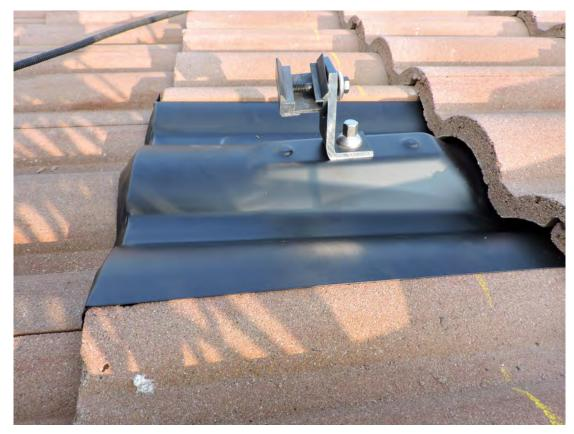
Ultra Rail W Tile Replacement Solution, Installed
