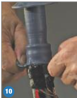
10. Fold down the skirt over the mastic to seal the cable entrance.
