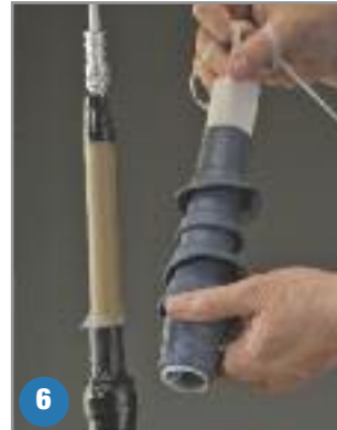
6. Pull the loose end of the core cord until the core is even with the end of the termination housing.
