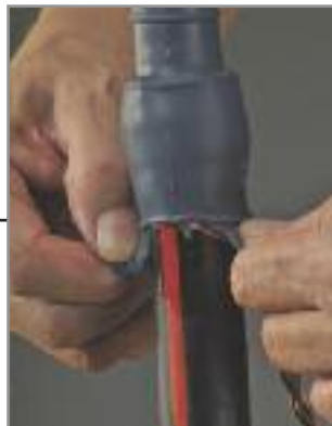
8. Shrink into place by unwinding the removable core.
