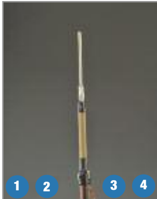
1. Train the cable into position and cut to length. Using standard practices, cut back the cable jacket, metallic shield, semi-conductive shield and cable insulation, exposing the conductor.
