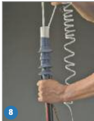
8. Shrink into place by unwinding the removable core.
