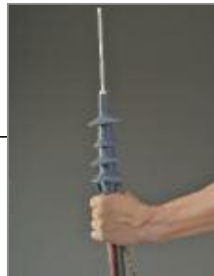
6. Pull the loose end of the core cord until the core is even with the end of the termination housing.
