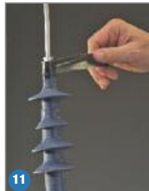
11. Seal the top of the terminator at the connector area with silicone tape.
