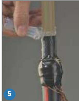
5. Apply a liberal bead of silicone lubricant to the semi-conshield step.
