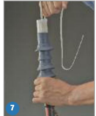
7. Position the terminator onto the cable.
