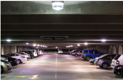
Before: Metal Halide Lighting
