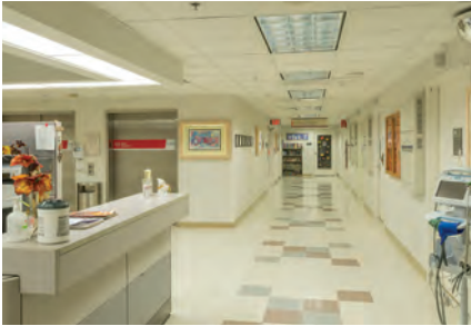
Before: Fluorescent Lighting
