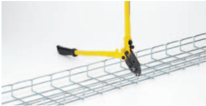
1 Face tray up. Slide cutter next to vertical wire and cut.
