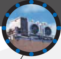
HVAC energy controls
