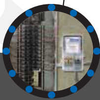
Whole home surge protection
