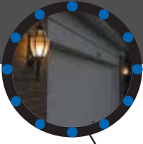
Garage lighting controls
