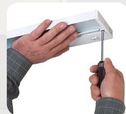
Step 3 Mount fixture to cabinet bottom using captive mounting screws
