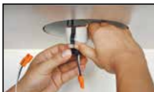
STEP 1: Twist Adaptor into socket.
