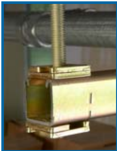
New method using Trapnut® Strut Fastener.
