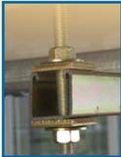
Standard method using nuts and washers.
