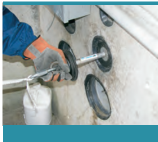
Attach pulling tape to carrier and insert carrier into pipe.
