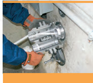
Install threaded adapter into conduit and assemble split winch line blower body.
