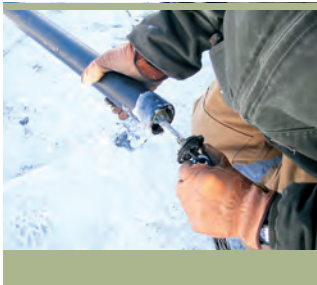
Attach winch line to carrier and insert carrier into pipe.
