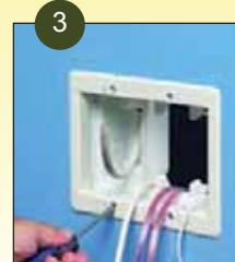
3 Tighten mounting wing screws to pull the box securely against the wall board. See Photo B.
