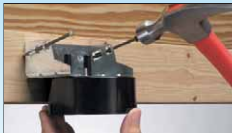
Nails to SINGLE JOIST
