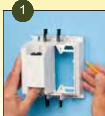
1 Using box, without trim plate as a template, mark location. Cut hole.
