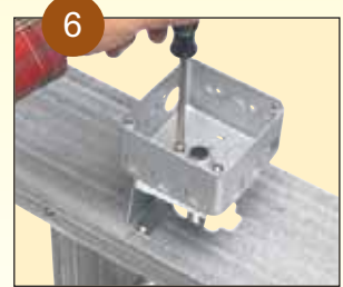
Attach 4x4 metal box to the stand-off bracket with screws (not provided) through pre-drilled holes in bracket.
