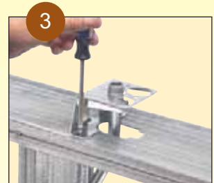
Attach B44 stand-off bracket to metal stud through holes in base.
