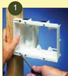
1 Attach box to stud. Use tabs for proper positioning of box depth. See 2.
