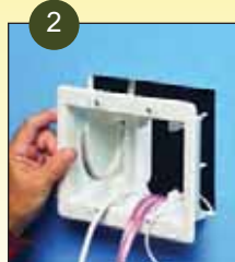
2 Attach trim plate to box. See Photo B. Pull wire/cables. Install box assembly in opening.
