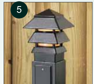
5 Install pagoda light to post with locknut inside the top of the post. Wire fixture.
