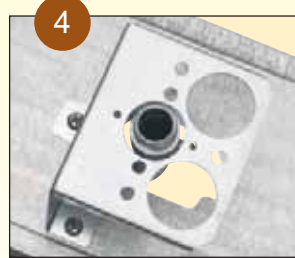
EMT "floats" in clearance hole to assure proper bonding between box and fitting.
