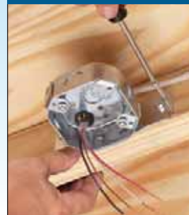
FBS415S/FBS420S Mount on SIDE of Joist
