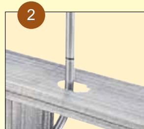
EMT marked and ready to cut.
