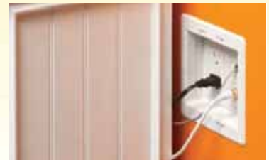
Finished Installed Shot.
