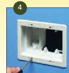
4 Tighten mounting wing screws to pull the box securely against the wall board. See Photo B.
