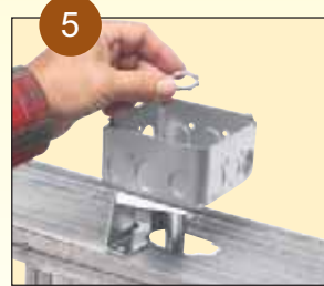
Install locknut on EMT fitting.
