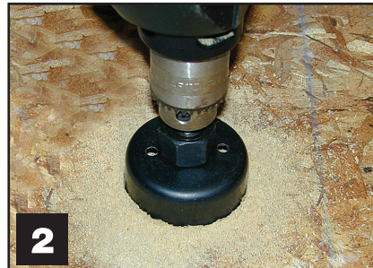
Figure 2 - Drill hole in floor using a hole saw.
