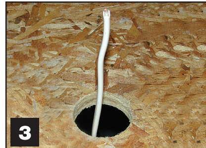
Figure 3 - Pull NM Cable through floor.
