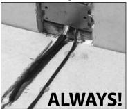
Always <u>completely</u> embed the factory splice and all heating wire in mortar. NEVER bend the splice or place any part of it in the wall or through the floor.
