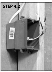
Install an extra-deep single-gang box if connecting one or two cables box with a single-gang mud ring cover if connecting three cables, because the extra room is needed for the wire, wire nuts, and control.
