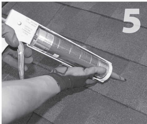
5 Clean off any sawdust, and fill hole with sealant compatible with roofing materials.
