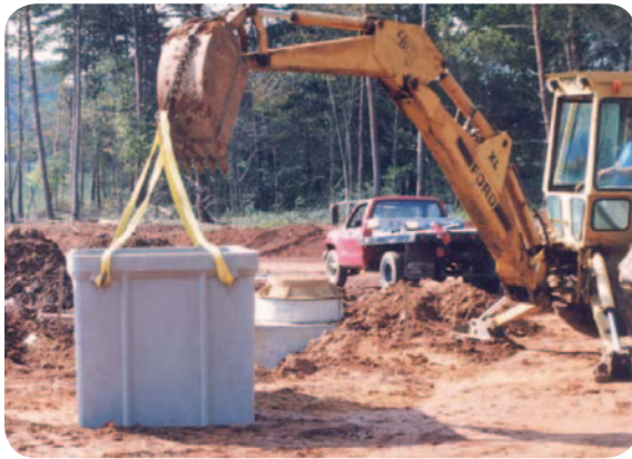
Lift and position enclosure with backhoe.
