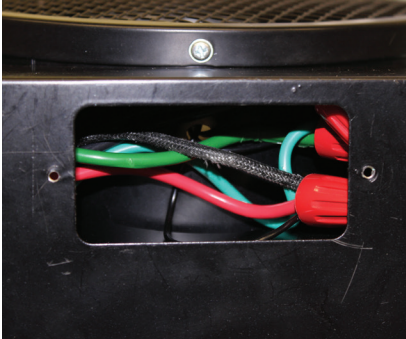
Figure 14: Wire connections carefully pushed into wiring compartment.
