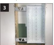
Attach brackets at the top and bottom of the enclosure.
