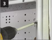
Install frame and lid using the provided No.8 screws.
