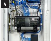
Recommended load 5lbs (2.27kg) Place in heavier equipment first.
