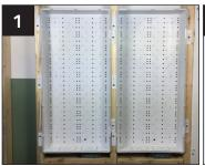
Place enclosures between studs side-by-side.
