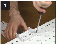
Attach the bracket at the back using the screws provided.
