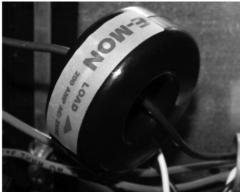
Fig. 6. Solid-core Current Sensor.
