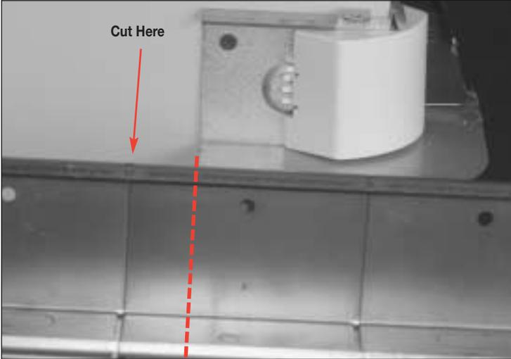
**Use scores on DS4000 Raceway Base to make cuts** – Snip where shown and bend along scored line to break.
